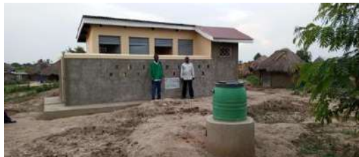
Figure 3.1: The LC1 chairman and his Vice posing in front of newly constructed pit Latrine in Kabolwa trading centre.
